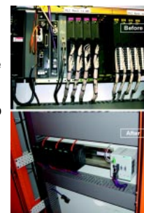
Above: the old wiring; below: the new!
